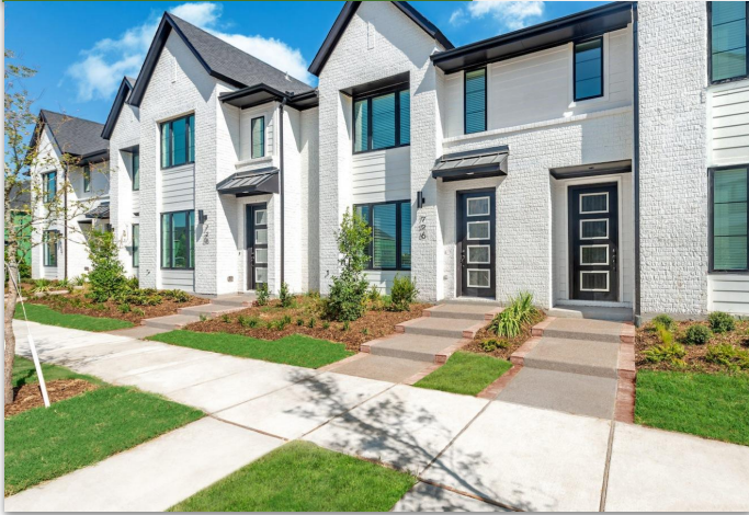
STREET LIGHTS 32 Two-Story Townhomes
